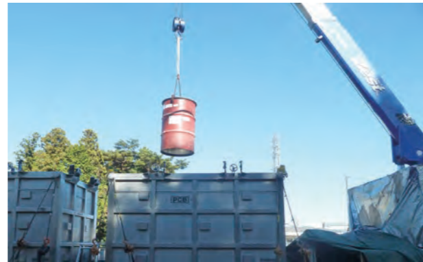
Up-close look of PCB waste removal
